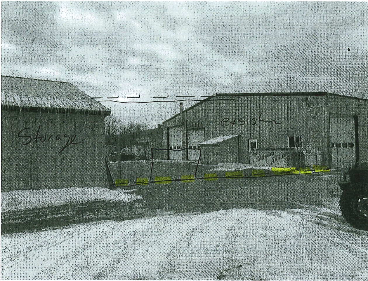
Addition on back of building
