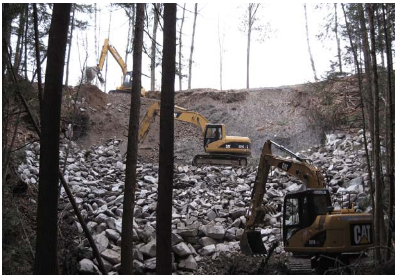
Repairing wash-out along Goldthwaite Road
