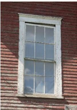
This south-facing window is one of many needing repair to seal the exterior of the historic fire house from weather, now that the building has been stabilized.
