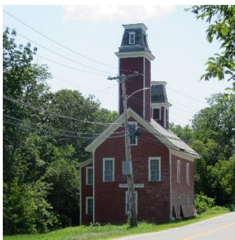
On the north side of the Yosemite Firehouse, a new door – with handicapped ramp entrance – will be cut on the first floor to the left of the existing window, which looks into the hose tower.
