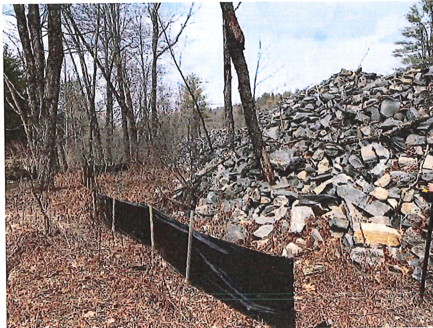
Photo 2: Fill encroaching into floodplain, trees growing up through fill show location of previous break in slope.
