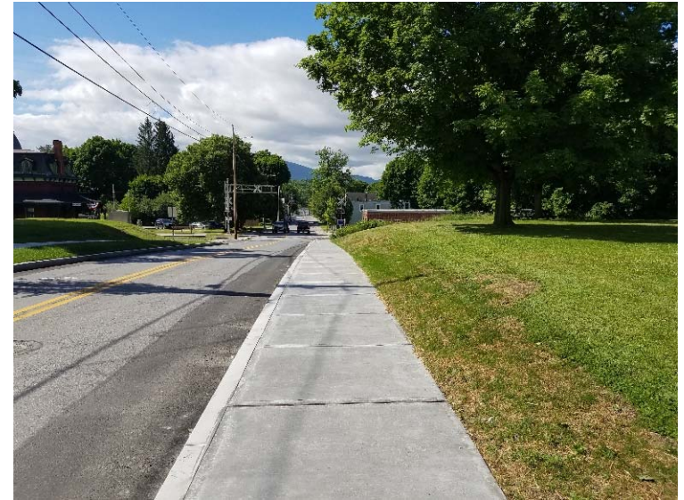
Sidewalk w/ Curb
